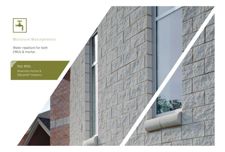
RainBloc® GP is a patented technology that can be added to mortar or concrete masonry block during the blending phase, which hinders water from penetrating the structure. This specially engineered formula creates a moisture barrier that will last the life of the building.
